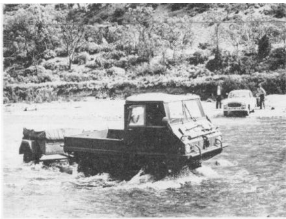
The high clearance of the Haflinger enables it to cross rock strewn river beds with up to 20 in. (508 mm) depth of water with minimum fuss.
